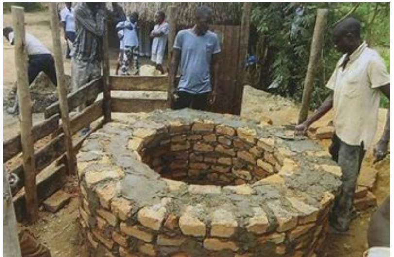
Example of what the well may look like when its finished.
